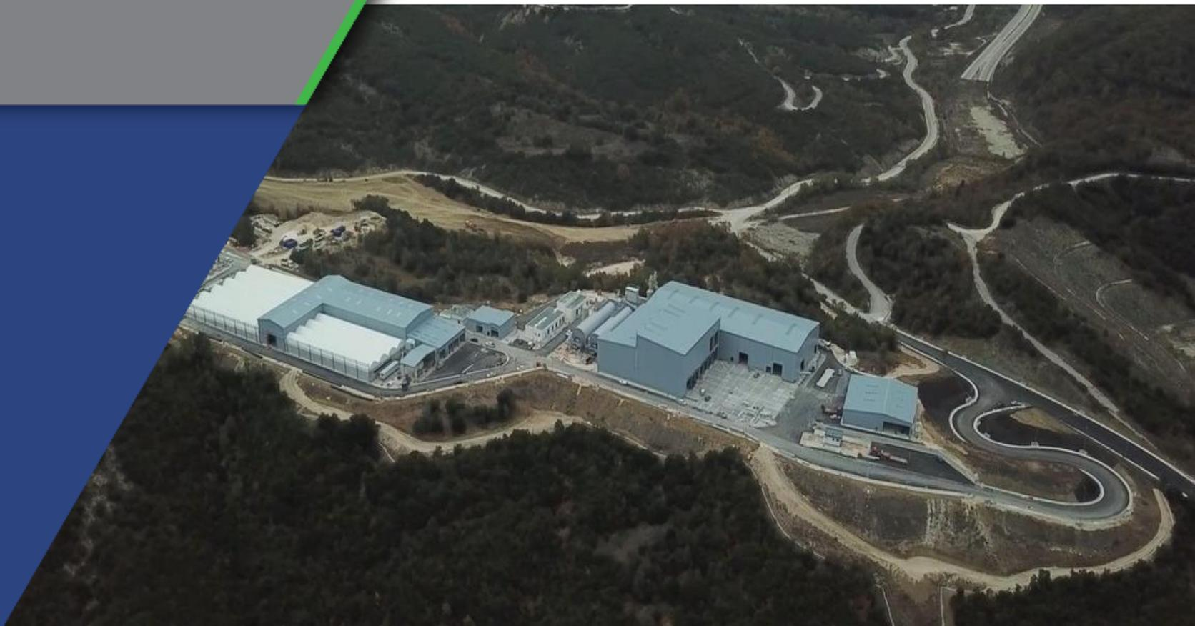
The project “Integrated Waste Management in the Region of Peloponnese” consists of three waste management facilities of a total capacity of 200.000 t/y and two transfer stations. Each waste management facility consists of a waste treatment facility and a landfill in which the treatment residue is disposed of.
